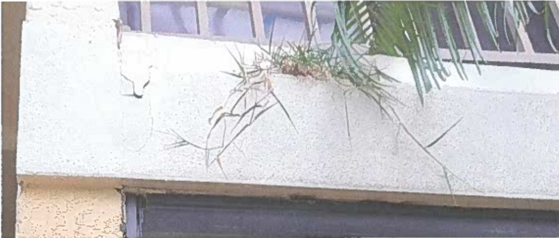
"B" crack on the exterior ledge. No rebar exposed. Rust stains are visible
