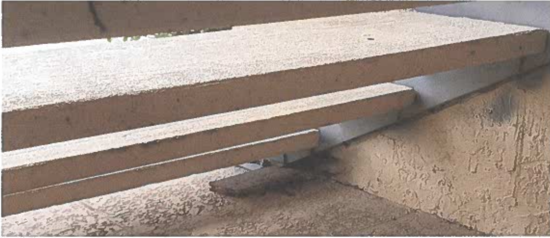
"B" crack on the exterior ledge. No rebar exposed. Rust stains are visible
